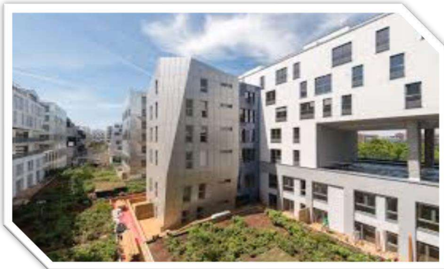
Figure 4 porosity on building exterior
