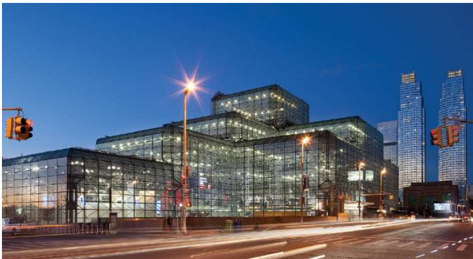
Figure 17 exterior view Source: - en.wikipedia.org
