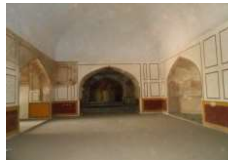
Figure 4: Basement Chambers towards West
