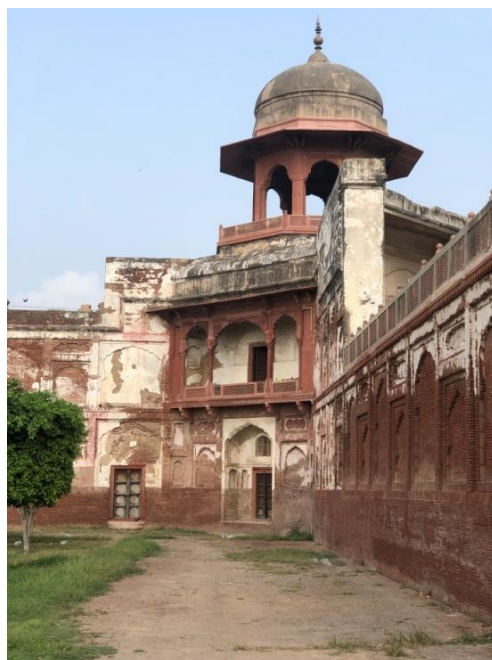
Figure 24 Octagonal Chamber over the Balcony
