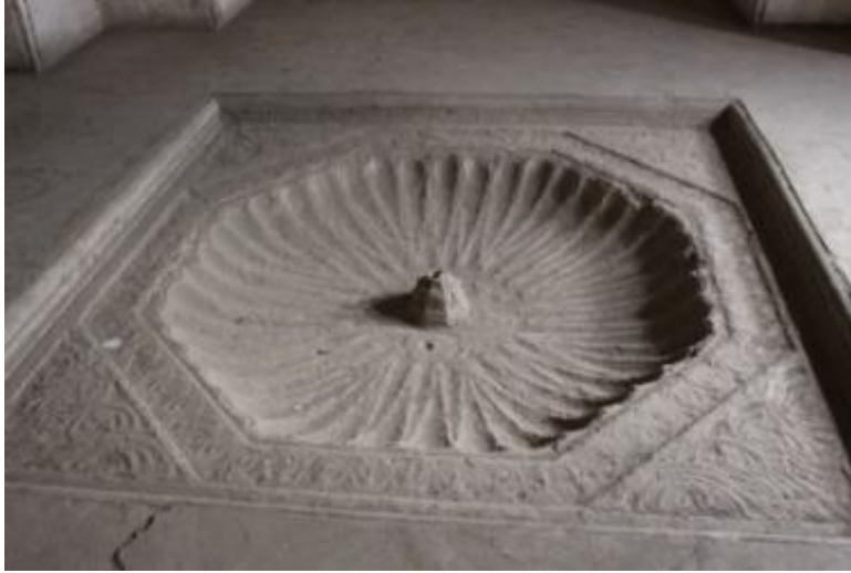
Figure 64: Picture Showing Finished Floor and Fountain Basin of Rakhtkhana
