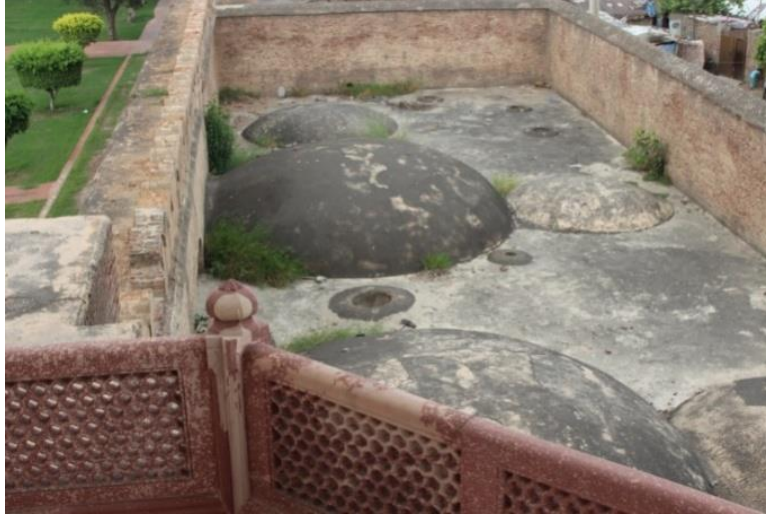
Figure 52: View of the Domes and Apertures in Roof
