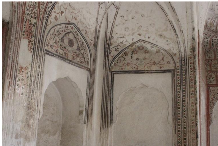
Figure 51: Pendentives and Squinches under the Domical Ceiling
