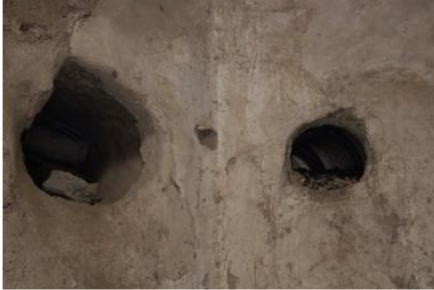
Figure 42: Terracotta Pipes Embedded in Walls
