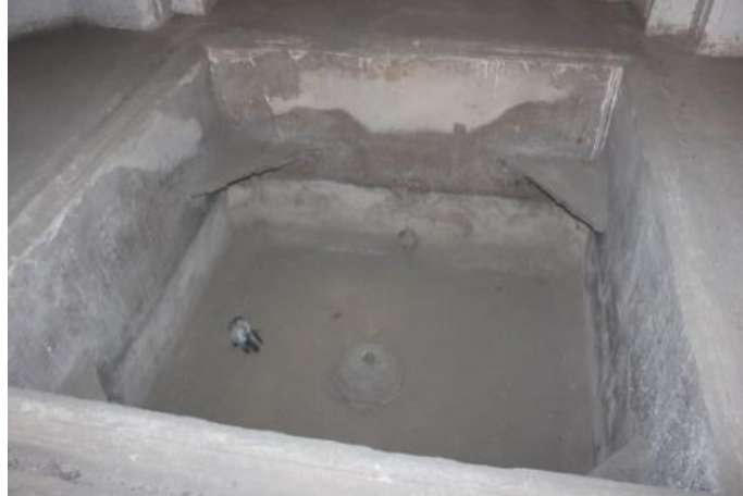
Figure 37: Square Tank of Eastern Part of Sardkhana
