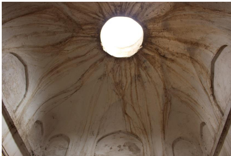
Figure 67: Aperture in the Centre of Dome to Invite Daylight
