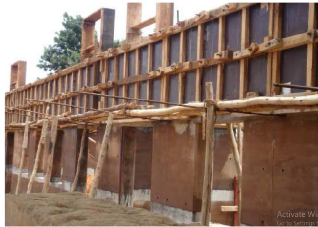
Figure 6 Rammed earth wall construction
