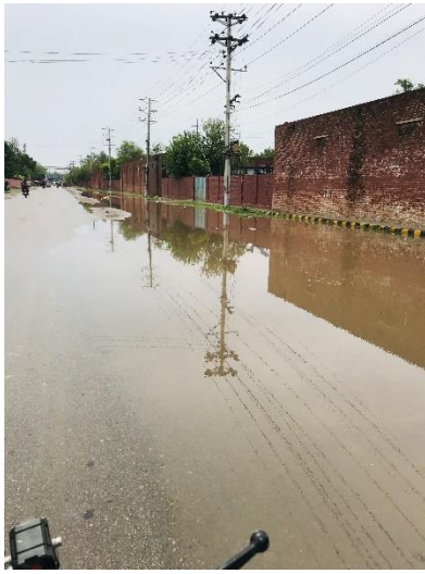
Figure 9. Katar Bund Road, Industrial Estate, Thokar
