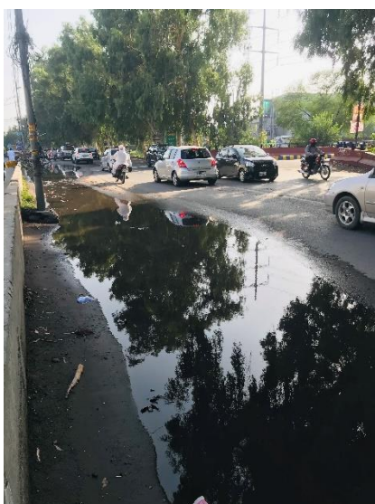
Figure 5. Canal Road Near Westwood Colony
